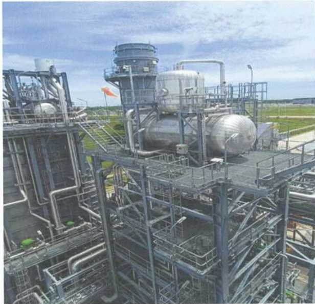
Feed Water Tank and Deaerator Drum
