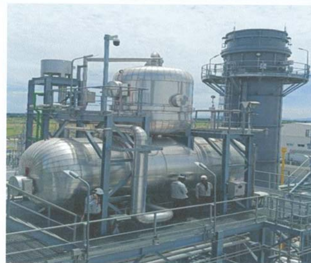
Feed Water Tank and Deaerator Drum
